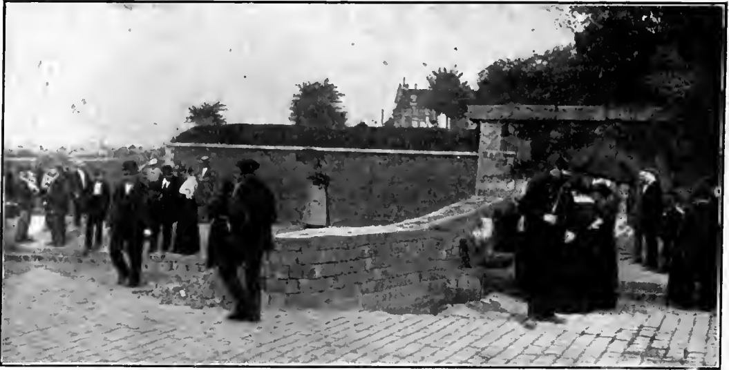
BUILDING A BARRICADE.
